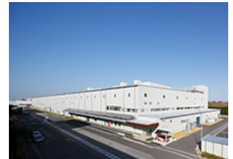
The waterborne paint Plant
